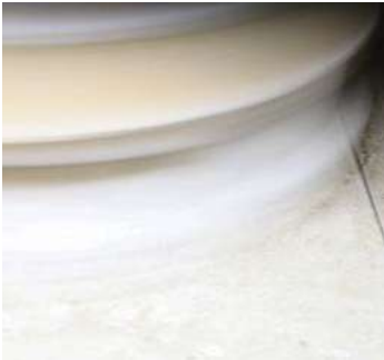
Treatment with «Easy-to-clean» application, which serves as protection of the high-gloss polish. Aplicación de la capa «Easy-to-clean» protectora del pulido alto brillo de la pieza.
